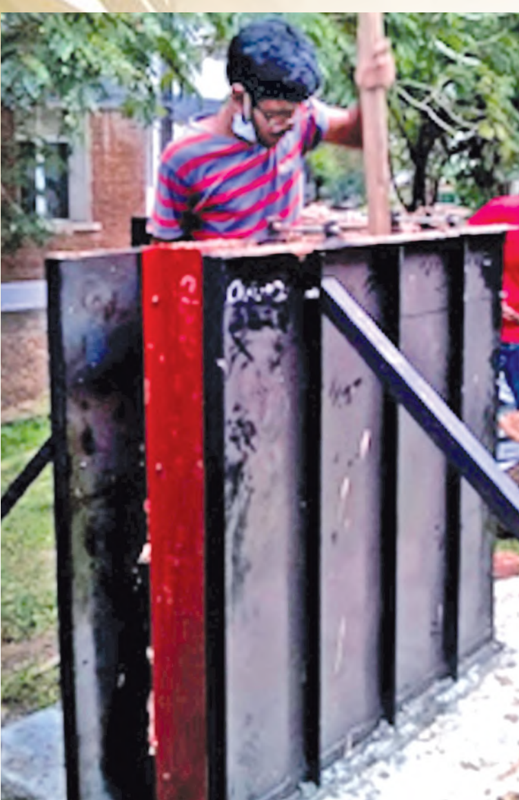
Figure 2: Assembling the formwork-Process of in-situ cast Mud-Concrete wall construction
